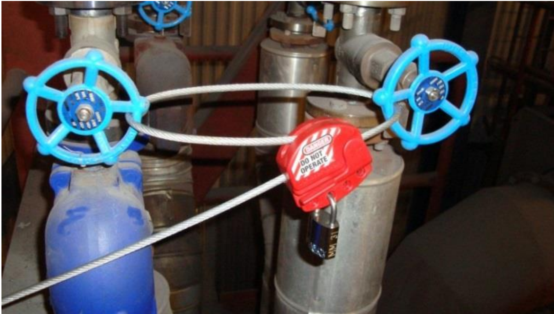
Picture 2. Cable with lock
