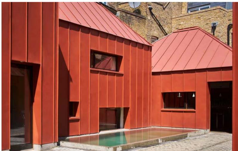
*GreenCoat PLX – a sustainable, highly formable colour coated steel for long strip roofing and façades that is workable at temperatures down to -15°C.*
